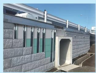
Foam-support construction method registered with NETIS.
