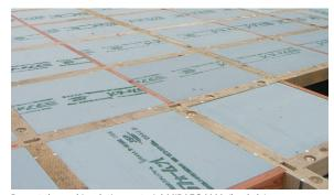
Pre-cut thermal insulation material MIRAFOAMA (lambda)
