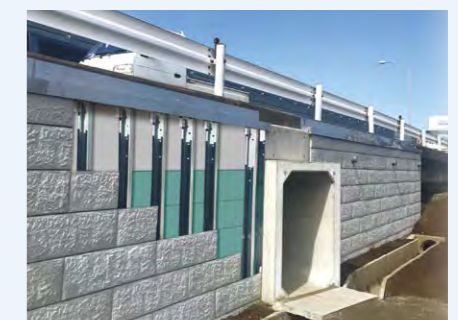
Foam Support Construction Method registered with NETIS.
