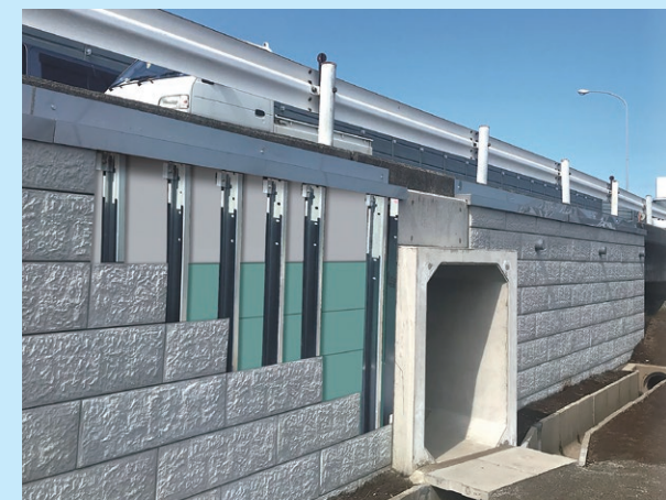
Foam-support construction method registered with NETIS.
